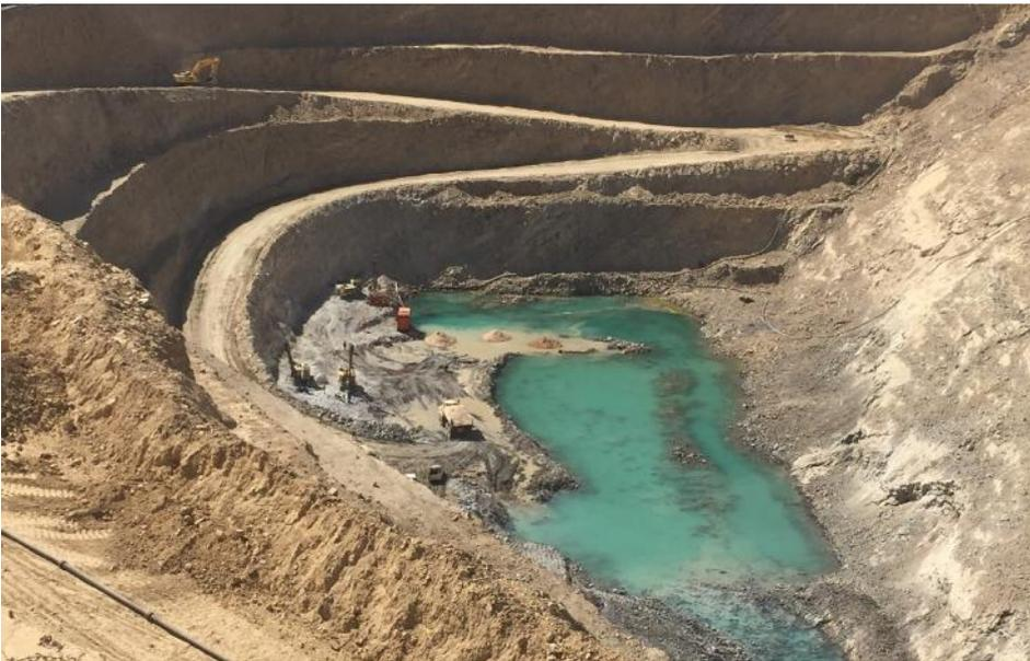
The open pit mine requires constant dewatering at a rate of about 800m<sup>3</sup>/h / hour.
