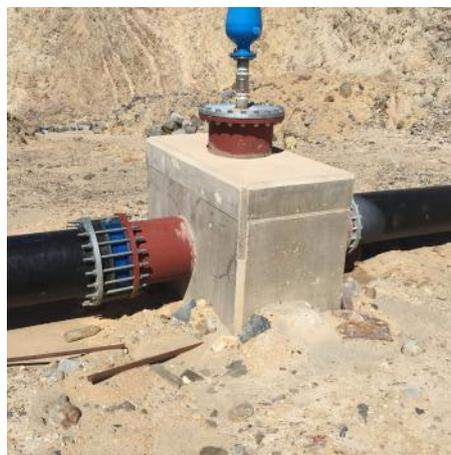
Thereafter the pipe followed a combined above- and below ground installation of another 2300m. The design had to take into consideration the rapidly varying pressure head, pipe transients (Water Hammer), air valve design and pipe restraints challenges in the pit and along the steep embankments.
