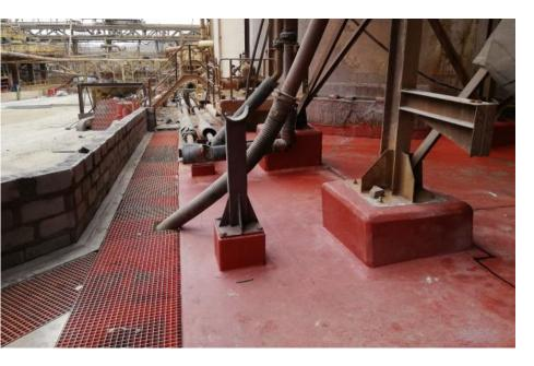
Rössing Uranium is one of the largest Uranium extraction mines near Arandis in Namibia. The project includes the structural investigation of the dilapidated concrete foundations and floor slab of their calcine reactor in their leach line, providing a durable solution and compiling the complete associated workpack for the project. Concrete portions that suffered sulfuric acid decay was removed, concrete repairs were done and acid proofing were installed to all concrete elements.
